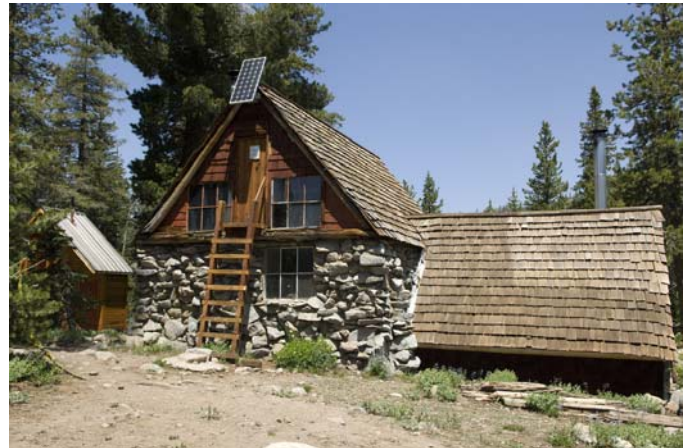
Peter Grubb Hut, built in 1938-39, has provided shelter for generations of skiers and snowshoers (photo by Joel Henner).
